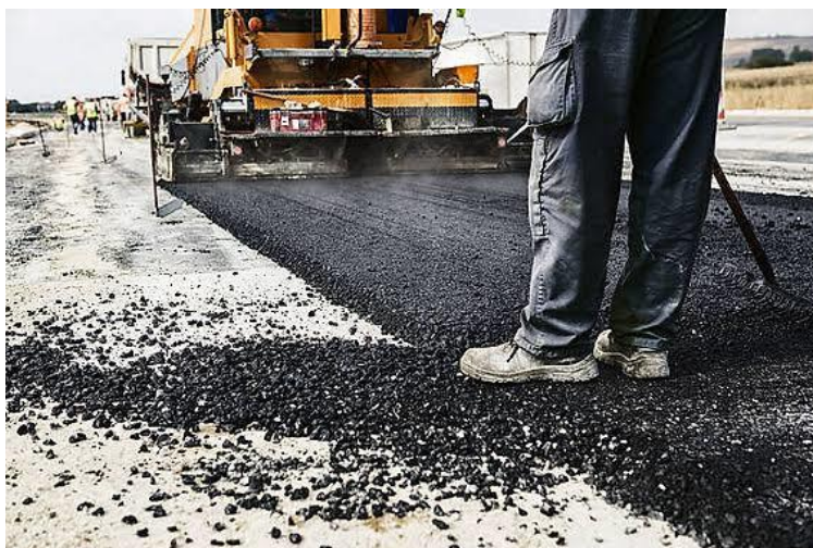
Plate 1: photo showing bitumen used in road construction.
